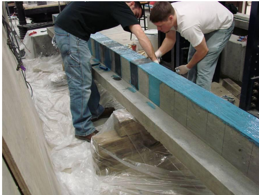
Figure 4.13 Application of CFRP U-Wraps
