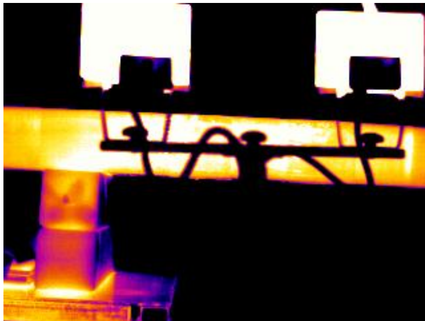
Figure 5.16 Infrared Thermograph at end of Warm-up Period
