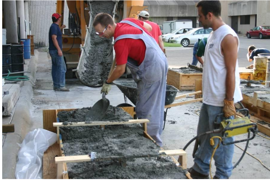
Figure 4.6 Casting of T-Specimens
