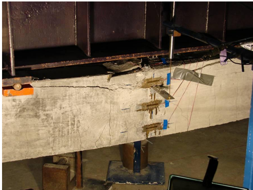
Figure 5.3 Control Beam R1 After Test
