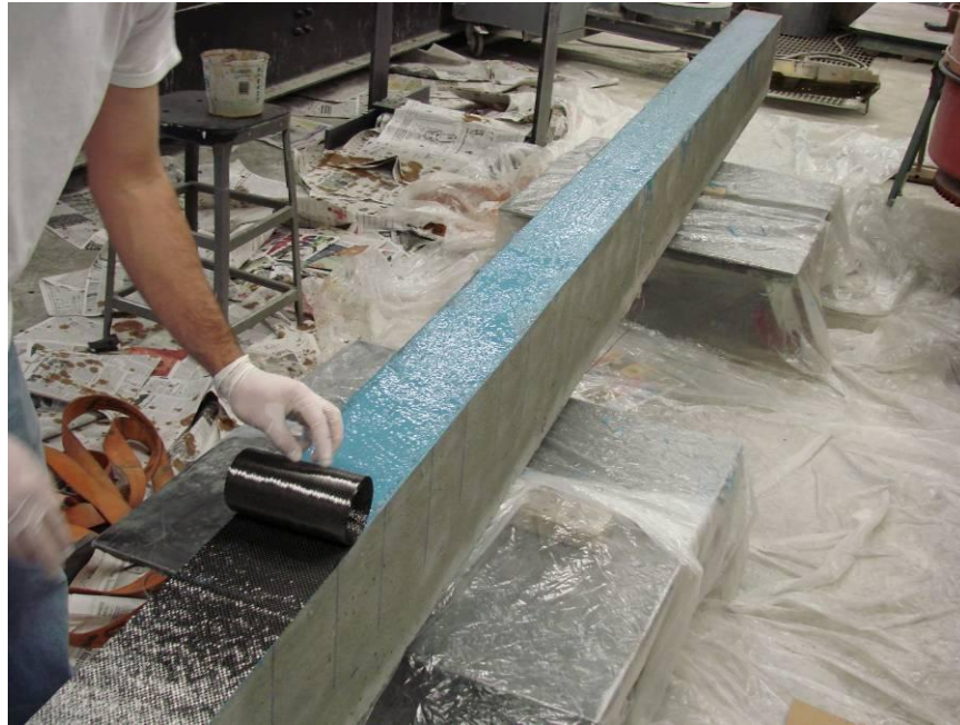
Figure 4.11 Application of First Layer of Flexural CFRP
