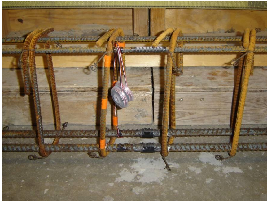
Figure 4.2 Strain Gages Applied to Mid-span of Flexural Steel Reinforcement
