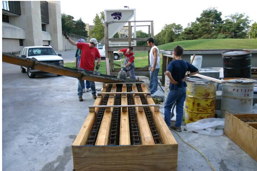
Figure 4.4 Casting of Rectangular Specimens
