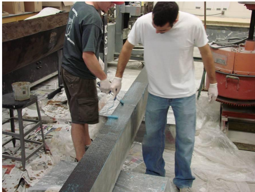
Figure 4.12 Saturating First Layer of Flexural CFRP
