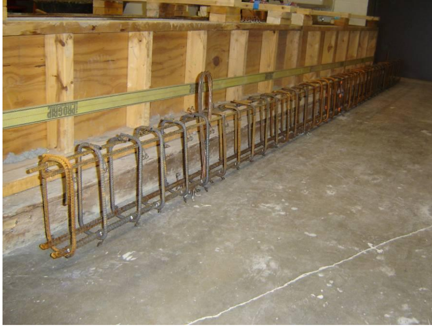
Figure 4.1 Rebar Cage Used for Rectangular Beams
