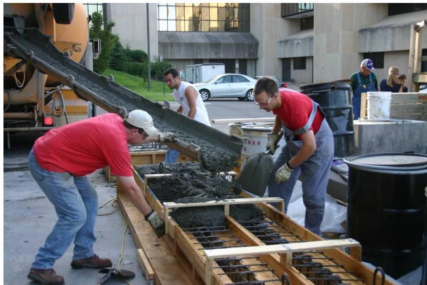
Figure 4.5 Casting of T-Specimens
