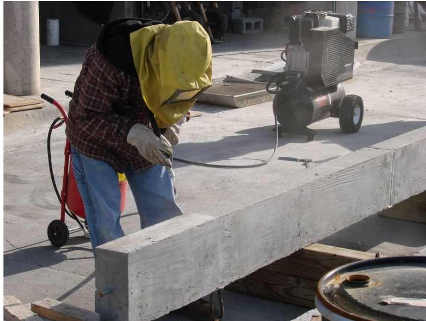
Figure 4.8 Sandblasting of Specimen Surface Prior to FRP Application
