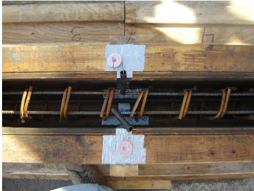
Figure 4.3 Rebar Cages Inserted into Formwork
